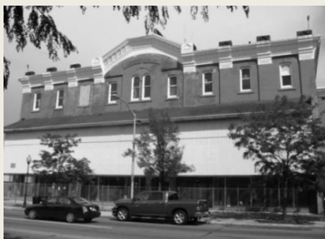
The G.G. Green Building, before (top) and after (right) restoration.
